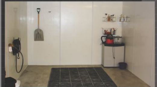
Wash bay is lined with extru tech on the walls and ceilings for easy clean up.
