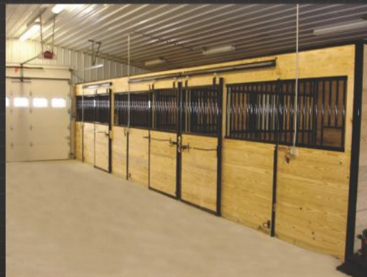
Custom horse stalls - tongue and groove southern yellow pine lumber, powder coated grills.
